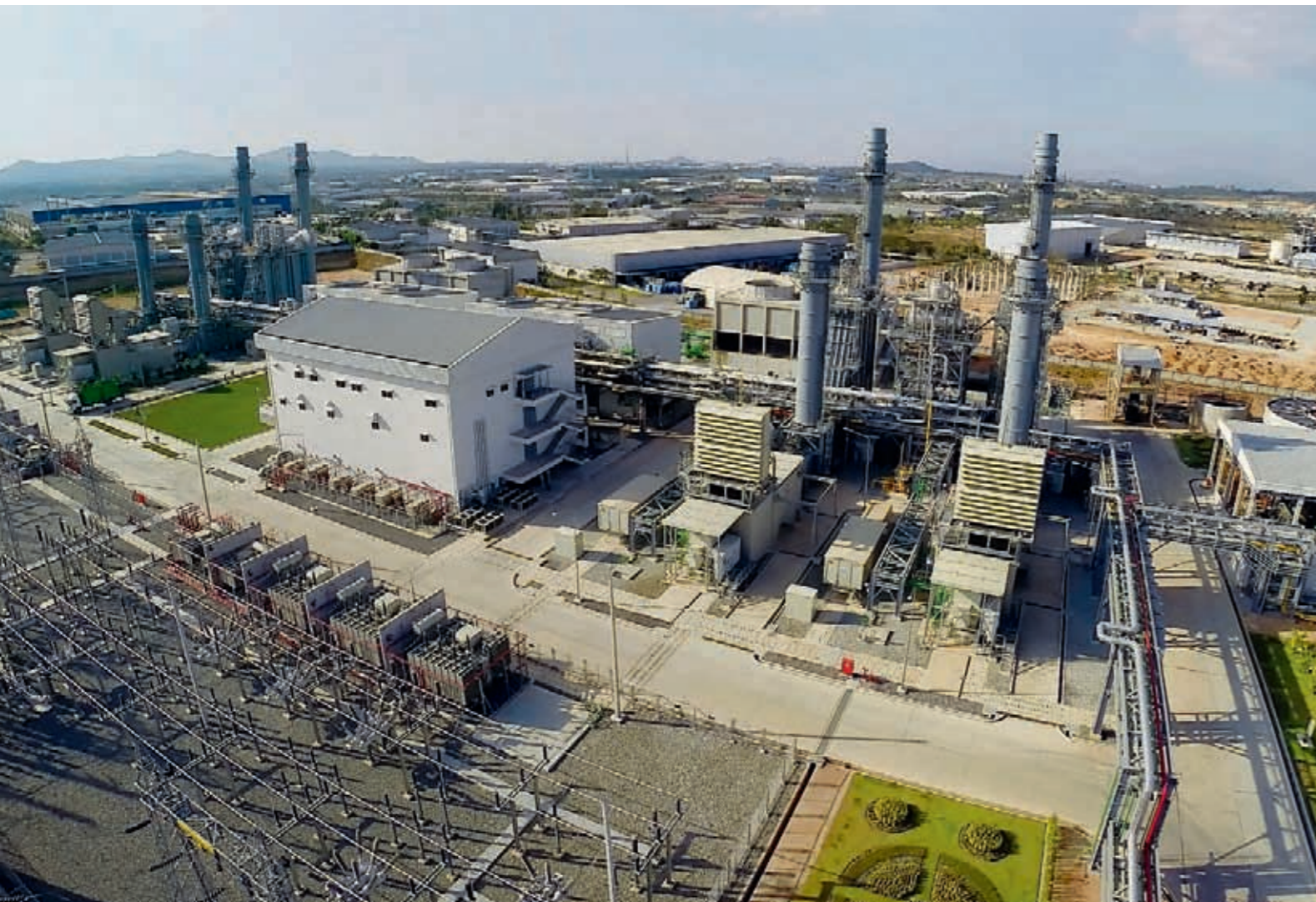
Four SGT-800 gas turbines and two SST-400 steam turbines at the new combined cycle power plant in Rayong's Amata City Industrial Estate create power for regional economic development.
