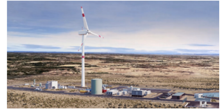
Haru Oni: the first large-scale plant to produce e-fuel from green hydrogen
