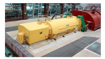
Our water-/hydrogen-cooled generators provide the flexibility and durability to operate in today's fluctuating grid environment. They can be coupled to other OEM turbines and meet environmental requirements as well as your individual needs.
