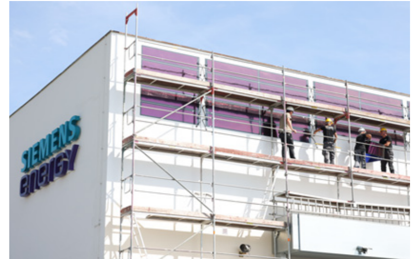
Installation of flexible photovoltaic film modules on Nuremberg power transformer factory.
