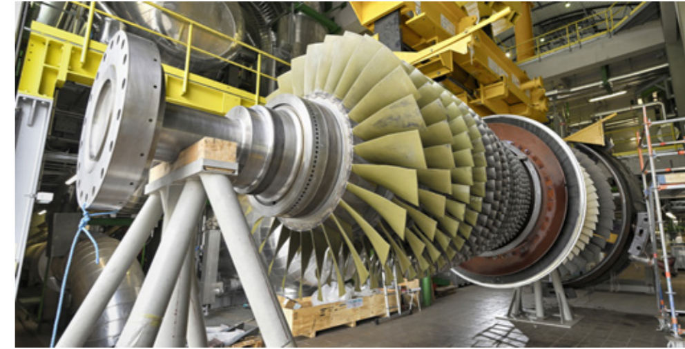
Gas turbine maintenance at the Donaustadt power plant.
