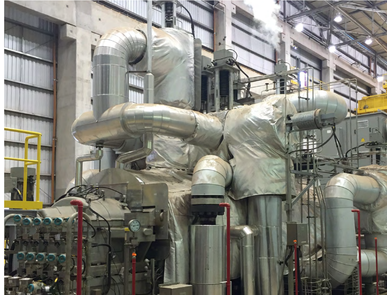
SST-800/500 Double-casing reheat solution
