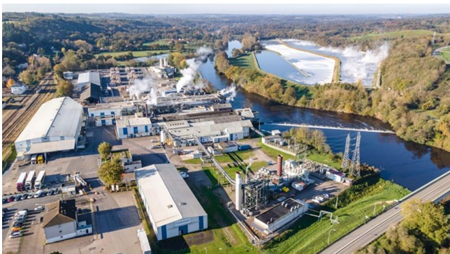
Figure 21: Smurfit Kappa SGT-400 Cogeneration plant in Saillat-sur-Vienne, France.
