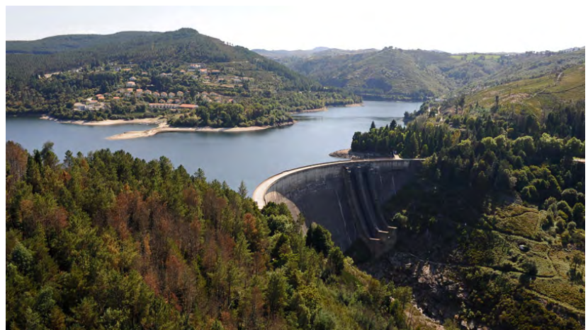
Fig. 3: Globally the most widely deployed bulk energy storage solution, pumped hydro is one of the most mature and proven technologies. It is based on a simple law of nature: gravity.
