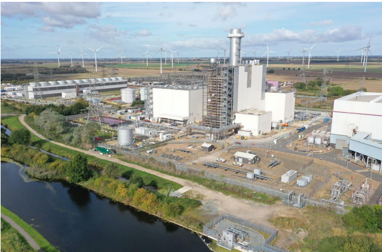
Keadby 2 is a new 840MW gas-fired power station in North Lincolnshire
