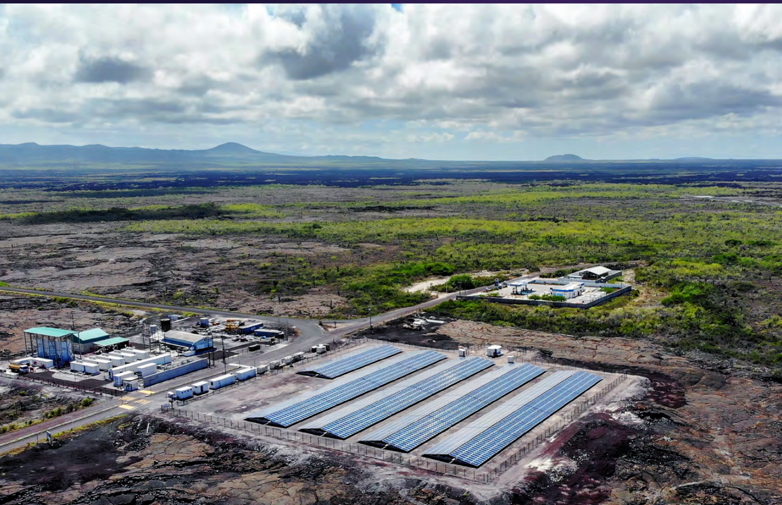
The Isabela Island Hybrid Power Plant on the Galapagos Island integrates solar and biofuel sources, an electrical energy storage system, and a smart hybrid control system
