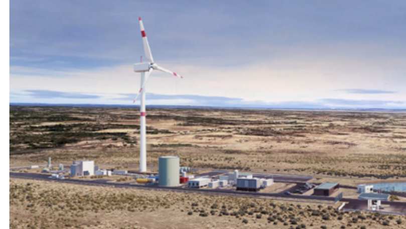
Haru Oni: the first large-scale plant to produce e-fuel from green hydrogen
