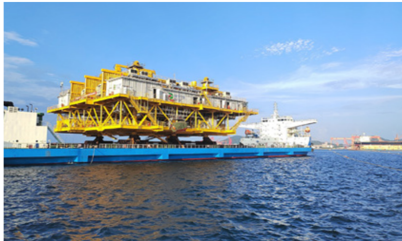
Transportation of the prefabricated modular offshore substation for installation.
