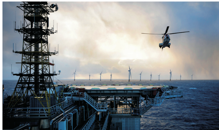
Hywind Tampen, pioneering floating offshore wind technology
