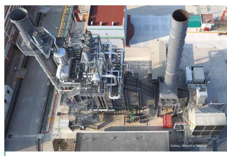
SGT-750 Industrial gas turbine Power generation: 39.8 MW(e) Mechanical drive: 34.0 – 41.0 MW Thanks to its wide fuel range capability and design features, the **SGT-700** is a perfect choice for several onshore applications: Industrial power generation, oil and gas power generation, and mechanical drive applications.
