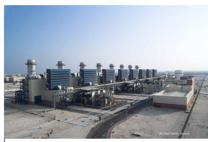
SGT5-2000E Heavy-duty gas turbine
