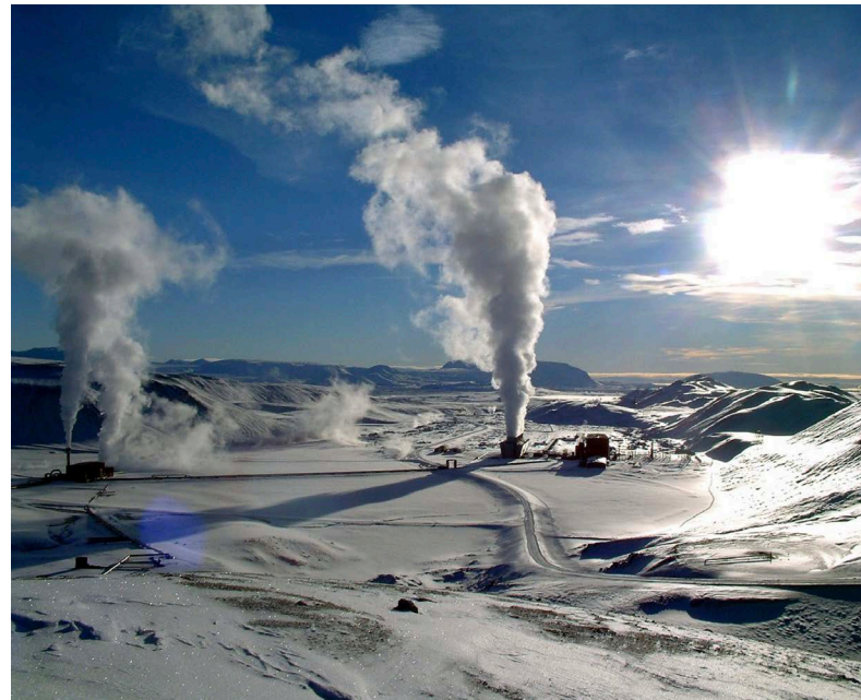
Krafla geothermal power station is located in the crater of the Krafla volcano in Iceland.
