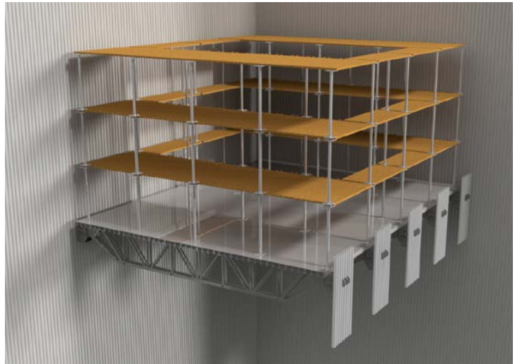
Boiler with service deck and scaffolding.
