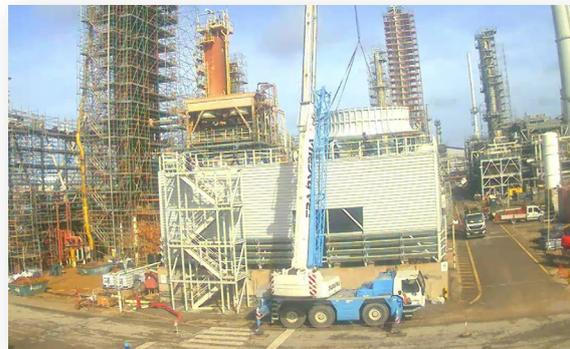
As the 21-day countdown continued, the focus transitioned from construction to the dismantling of the existing wooden tower. Days were dedicated to taking down the existing wooden cooling tower and then preparing the grounds for the installation of the new cooling system.
